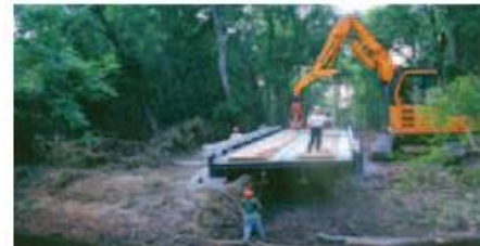
Figure 4-16. Example of a modular bridge with running planks. Photo: Big R Bridge
