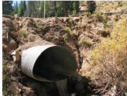
Figure 4-6. Culvert example 3. Photo: R.M. Edwards
