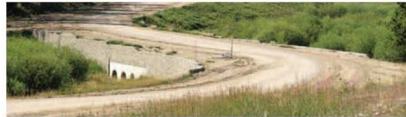
Figure 4-15. Example of a multiple culvert crossing with decorative retaining walls. Photo: R.M. Edwards
