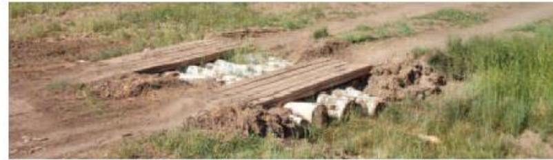
Figure 4-14. Example of low-tech solution for a temporary crossing using logs and lumber. Photo: Kelly Rogers
